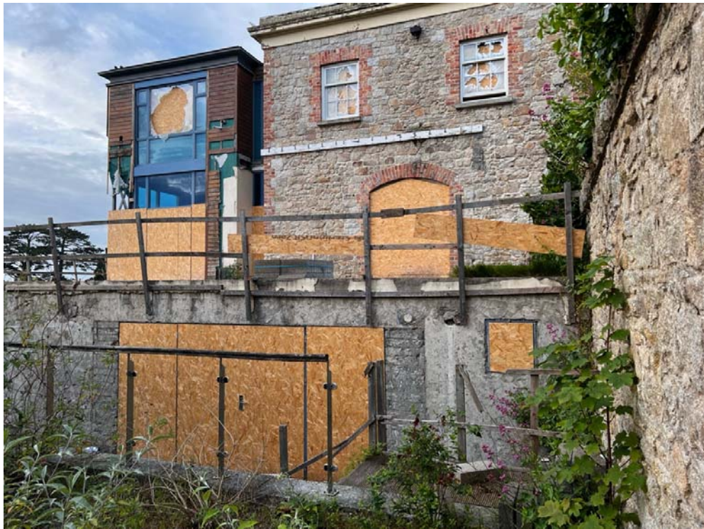
Plate 2. Western-facing side of main house
